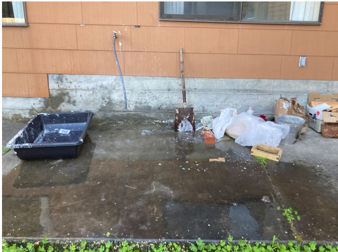
Concrete making station in backyard
